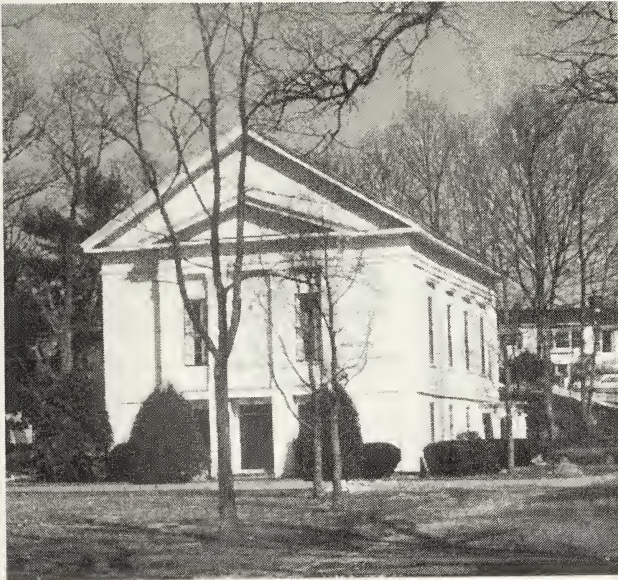
Parish House of the Congregational Church
